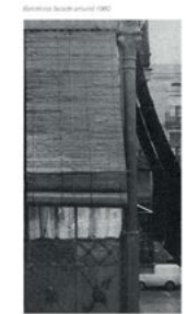
Barcelona facade around 1960
