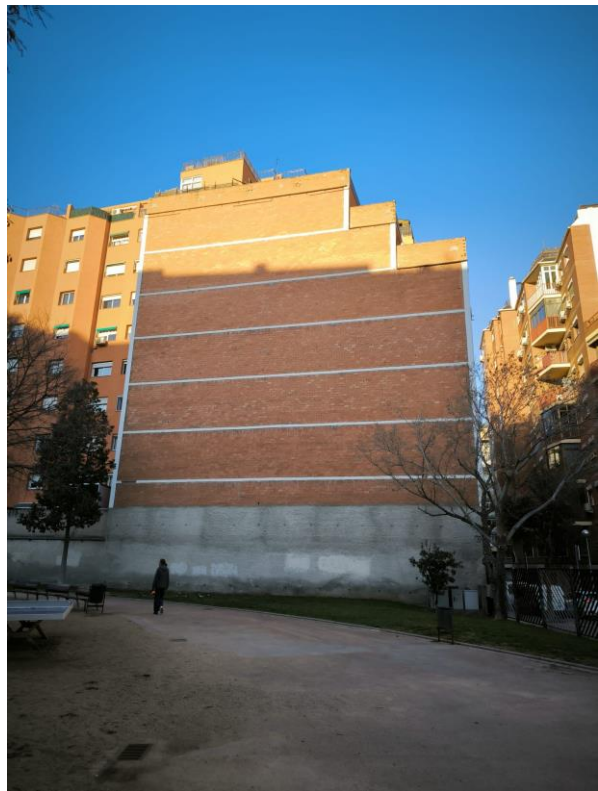
View of the party wall at C/ Quetzal 17-21
