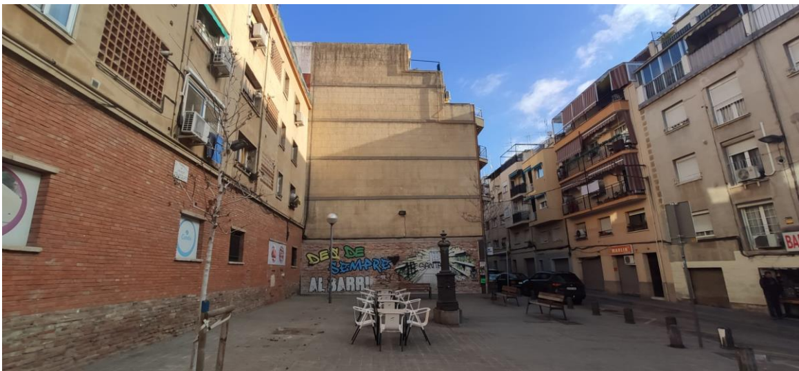
View of the party wall
