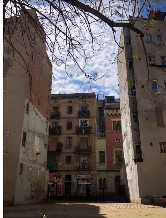
Walkway between C/ Hospital and the square
