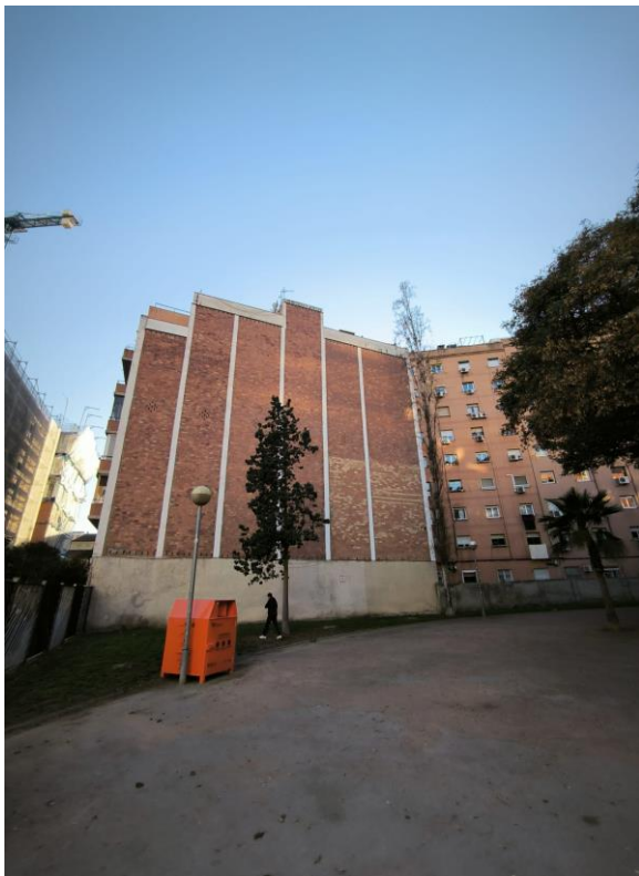
View of the party wall at C/ del Quetzal 5-7
