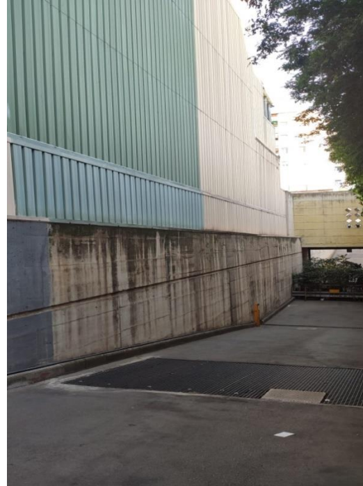
Walkway between party wall on Carrer del Rosselló and the Jardins
