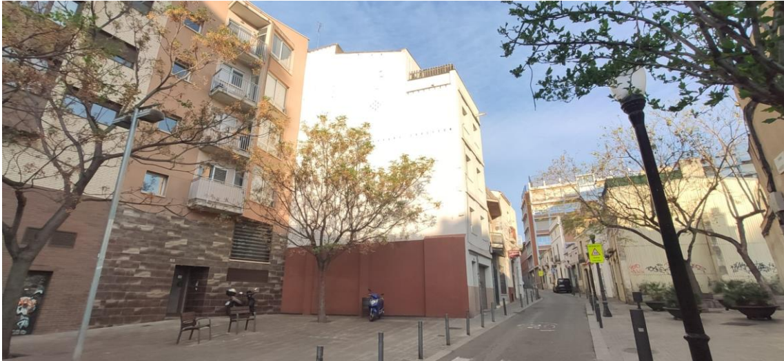
View of the party wall
