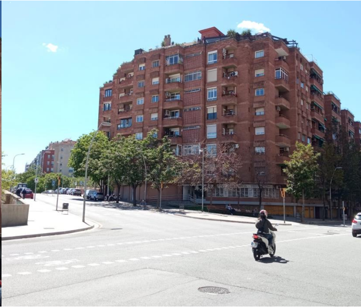
View of the façade
