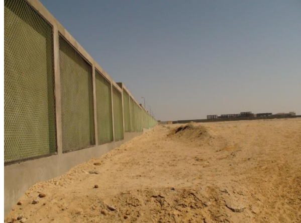
14 Site at the northeast
