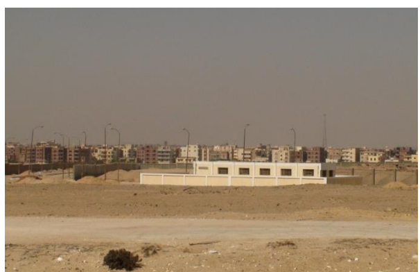
06 Electrical plant facing the site
