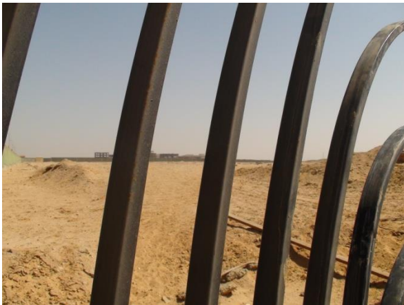
15 Fence detail at the northeast
