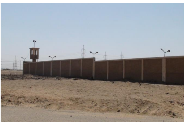
05 Electrical plant area
